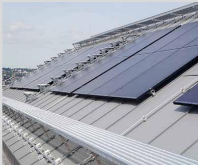
**GARDCO** safety rails can replace lifeline systems and safety posts. According to DIN 4426 guardrails should have priority to personal protective equipment (PPE) because they eliminate the fall hazard for all the workers on the roof simultaneously.
